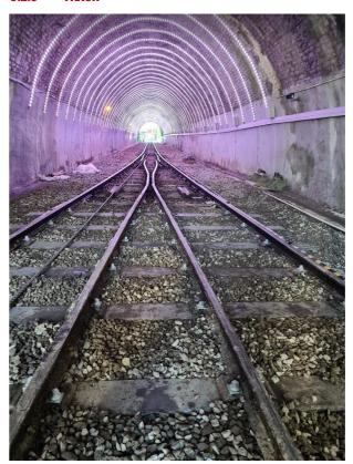
The track was installed in 1979, using second-hand rail supported by a mix of treated pine and hardwood sleepers. The sleepers are now over 40 years old, and the ones in exposed areas are due for replacement. This work will be prioritised and scheduled to be completed during our usual annual shutdown.
